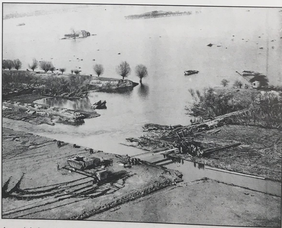
An aerial view of the Crowland North Barrier Bank breach.
