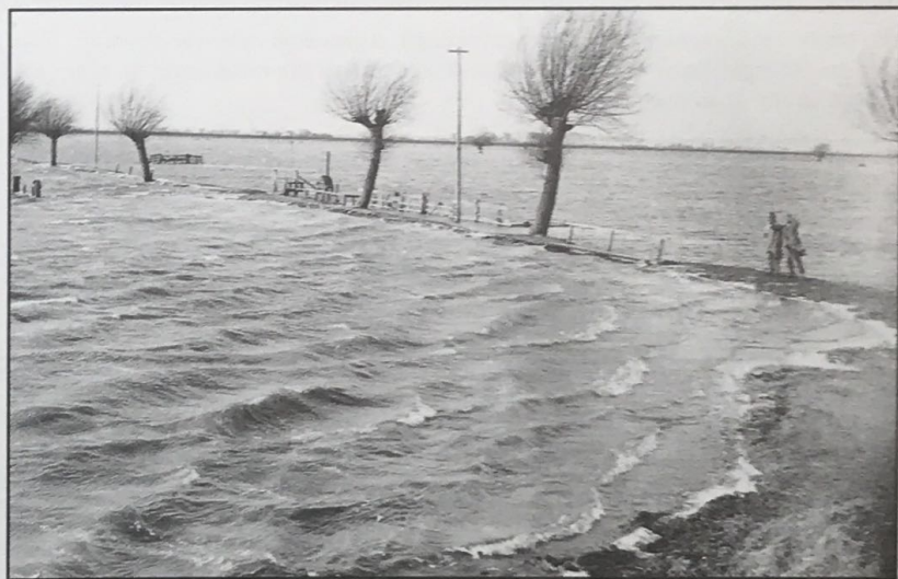
Gravel Causeway again, West Bank end. Compare this photograph with the second (early 1900s) picture of the water-carrier's cart on page 2. They were both taken from approximately the same spot.
