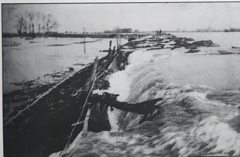
The River Welland above Fen Bridge (Deeping High Bank).
