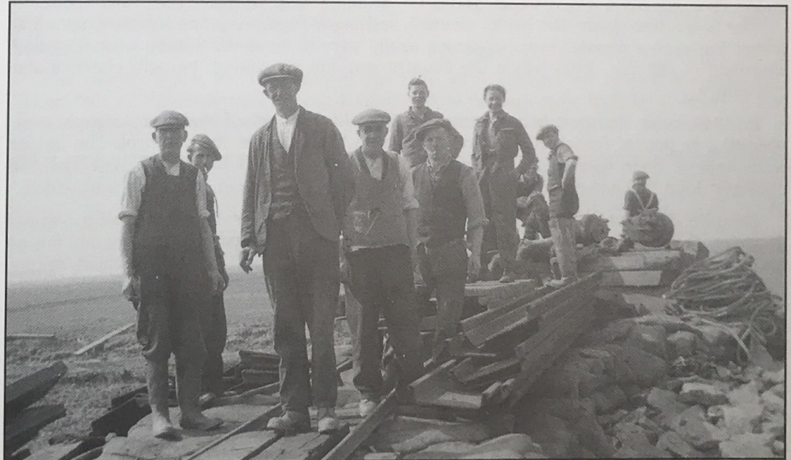
Two more groups of repair workers on the North Bank
