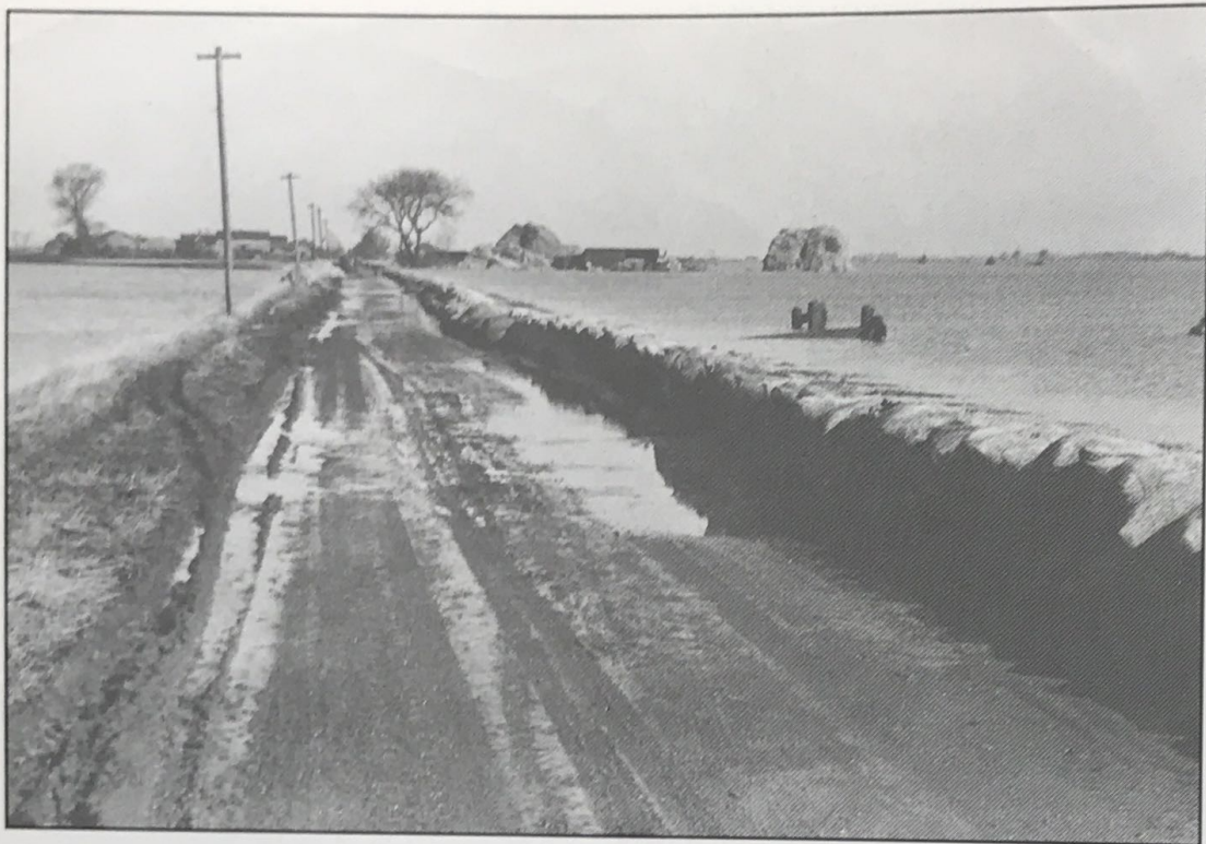
The scene on Speechley's Drove, Newborough, a few days after the flooding. Note the retaining wall of sand bags on the right, built to hold back the water so that the road could be kept open to traffic. Guns Farm can be seen in the distance.
