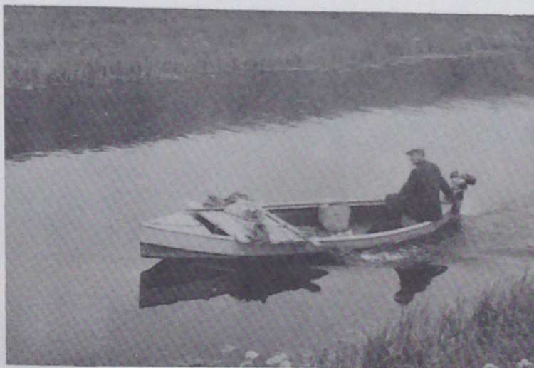
Copper Sulphate being applied to the South Drove Drain by trailing bags containing the Chemical through the water, 1965.
