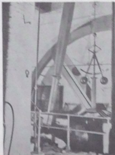
General view of Kesteven engine showing governor, part of fly-wheel, part of the connecting rod and a portion of the crank and bottom end bearing, taken through the archway connecting with adjacent engine house.
