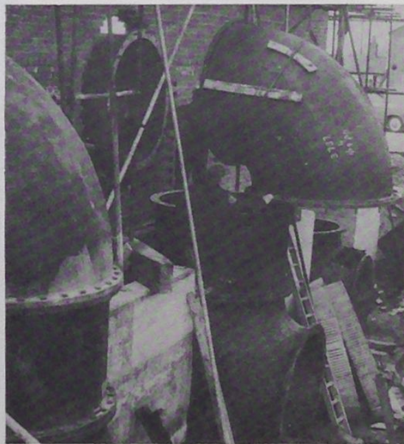
The discharge pipes of the pumps being installed.
