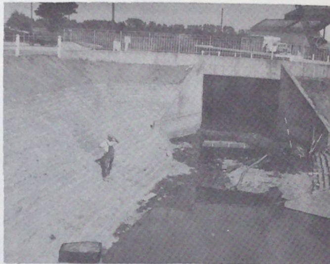
Stone pitching and concrete grouting of the outfall of the new pumps.
