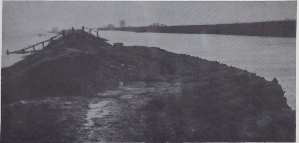
Sealing of the breach in the River Glen bank, 1947.
