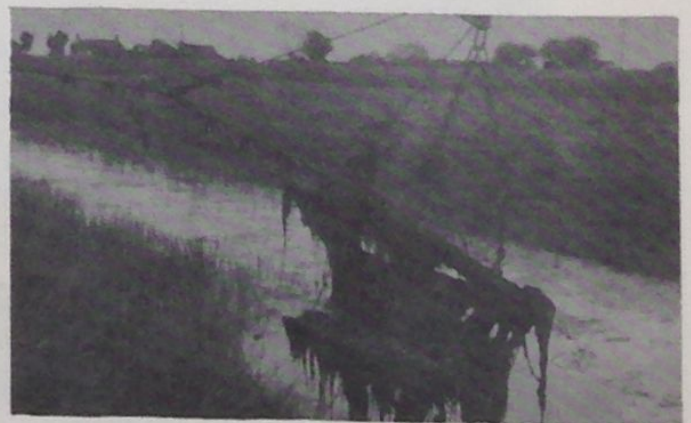
"Cott" being removed from the New River, Cowbit Wash, by Dragline Excavator.
