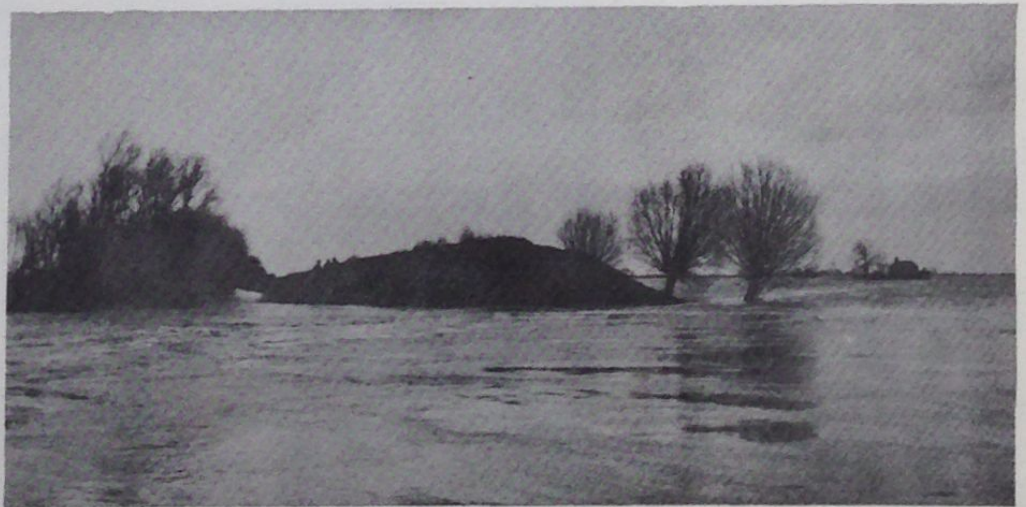
Breach in the North Level Barrier Bank, 1947.
