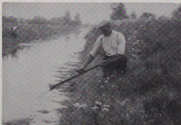
Roding of Counter Drain, 1965.
