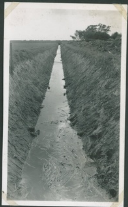
Dyke Completed. Note Cattle Destruction.
