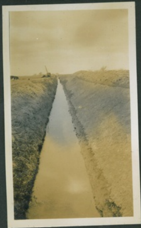
A STRAIGHT? WATER LINE.
