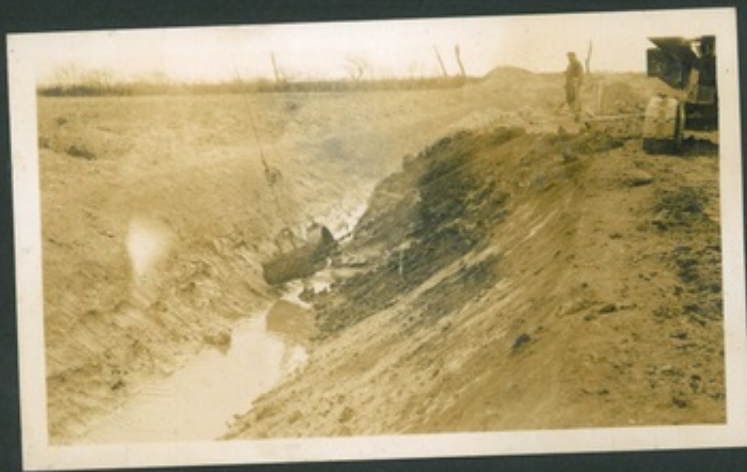
10 R.B. COLCHING S.W. BATTER TO COMPLETE JOB.
