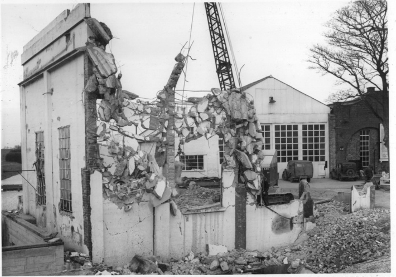
DEMOLITION OF BUREAU OF FIRE DEPARTMENT
