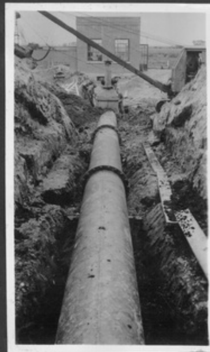
Works of laying pumps discharge pipes into River Glen.
