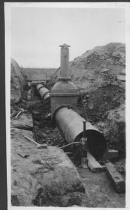
Works of laying pumps discharge pipes into River Glen.
