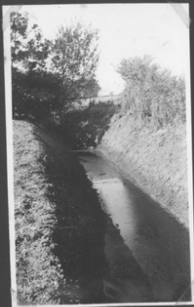
Cleansed by Hand Labour. End of Gravel Drain. Swinesmeadow Drain.
