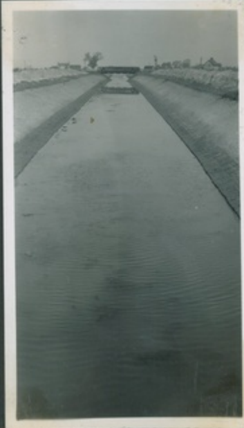
Downstream Horseshoe Bridge.
