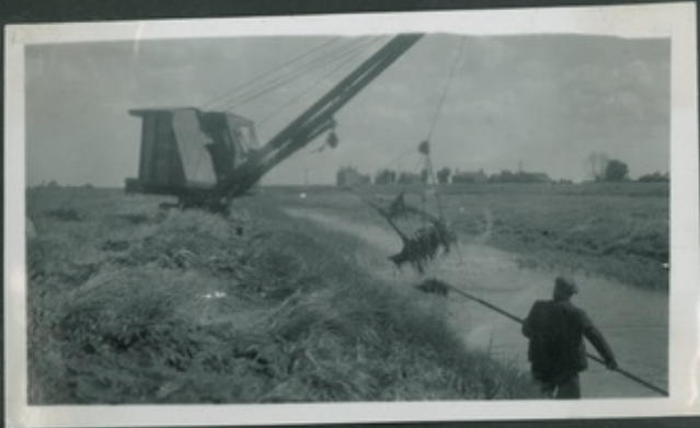
Cot Drag attached to Priestman Dragline, working in Cowbit Wash.
