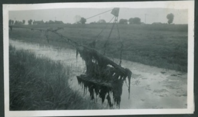
Cot Drag attached to Priestman Dragline, working in Cowbit Wash.
