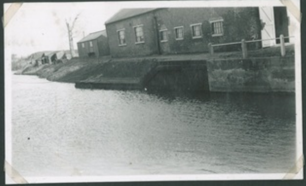
Job Completed. 5" x 5" Sheet Piling - 6" x 6" King Piles.
