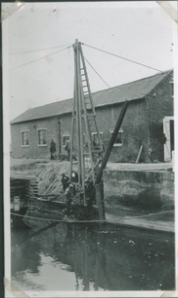
Driving 24'0" x 6" x 6" Oak King Pile with 50'0" Engine.
