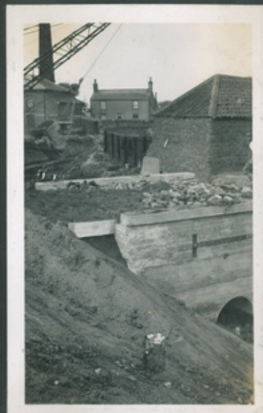
Refilling. Culvert completed.
