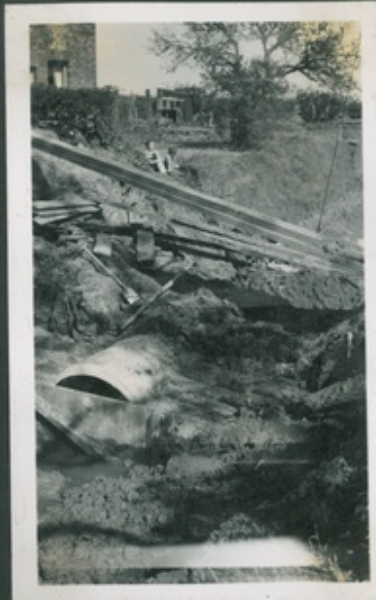
New 4'0" Dia. Tubes & concrete foundation.
