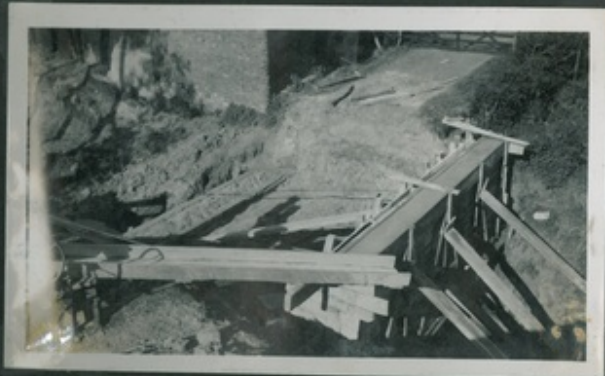
Shuttering for Walls.
