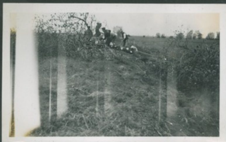
Tree felling in progress.
