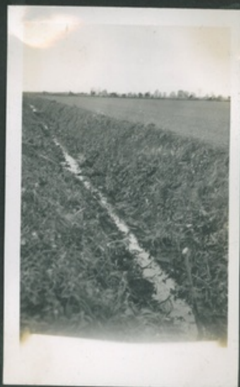
Dyke cleared of trees.
