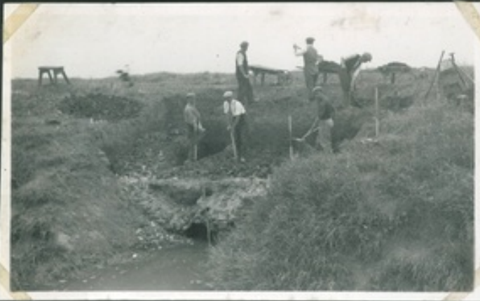
Commencement. Demolition of Existing Tunnel.
