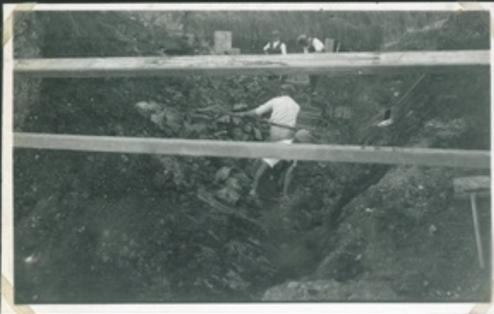
Excavation by Hand-Labour & Dragline.
