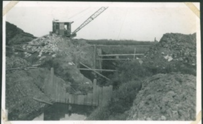
Road Closed. Excavation with 10 RB.
