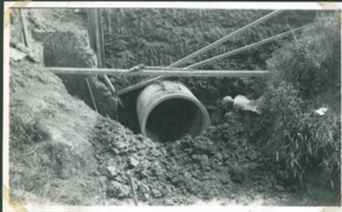
4'0" Dia. Tubes Laid. 5" Concrete Raft.
