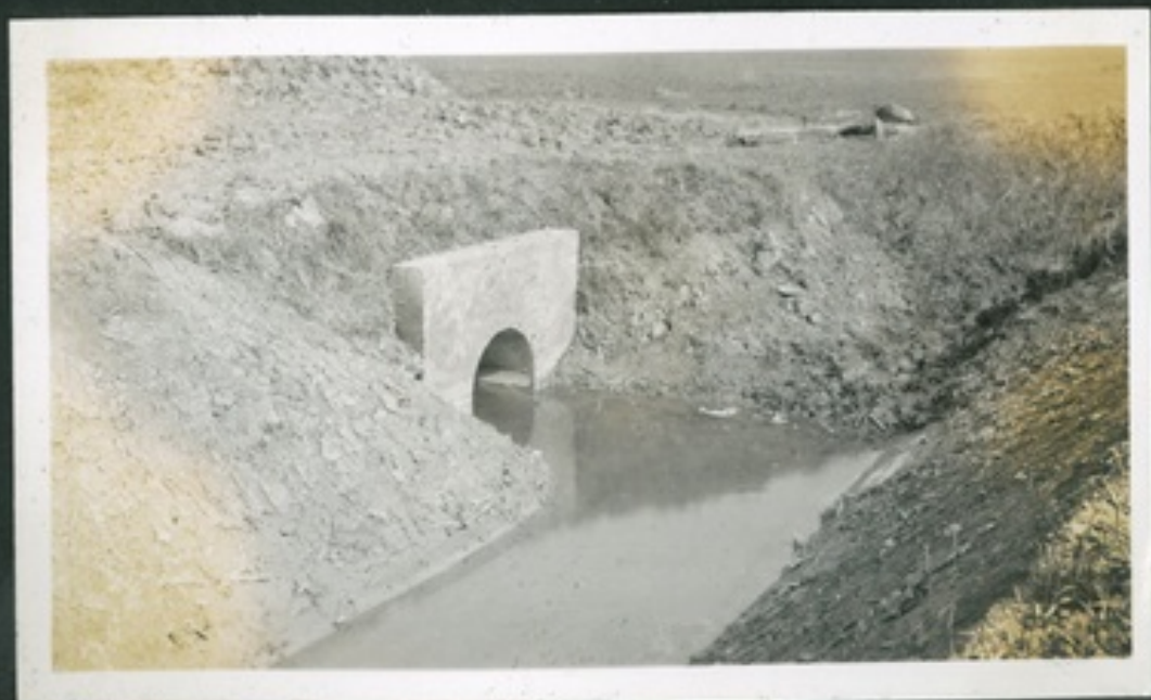
Small concrete heading wall on end of Culverts.
