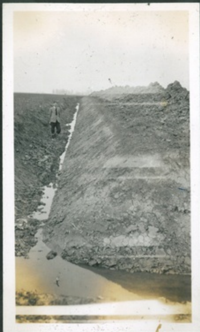
One side completed.
