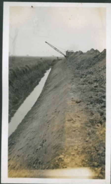
Working on one side.
