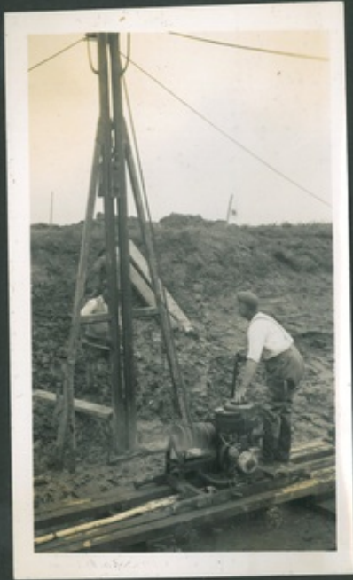
AUTOMATIC PILE DRIVER IN ACTION.
