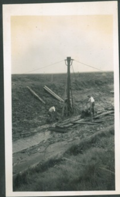
AUTOMATIC PILE DRIVER IN ACTION.
