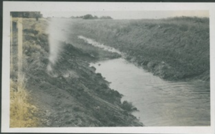
ROUGHING IN PROGRESS.
