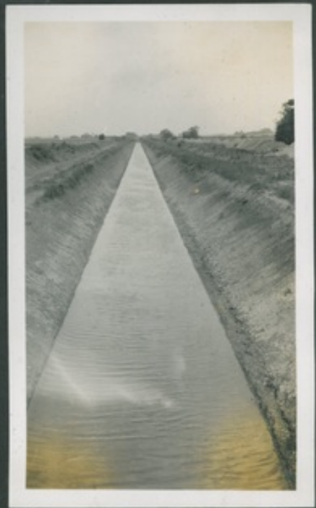
SECTION COMPLETED BETWEEN SOUTH DROVE & BARRON'S BRIDGE.
