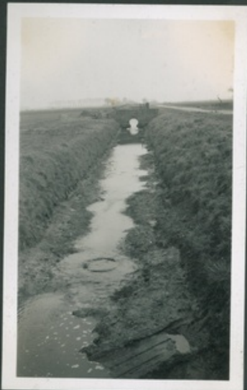
BEFORE WORK COMMENCED.
