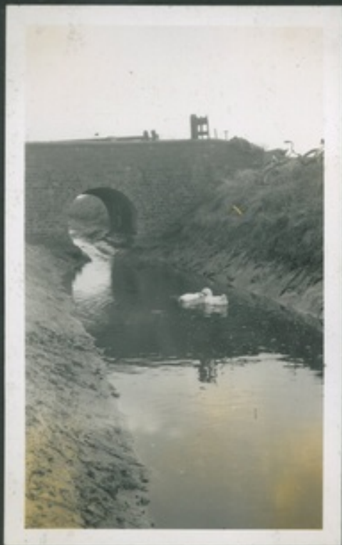
NOTE FLOW THROUGH TUNNEL!
