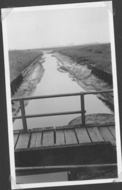
Low Water tidal-side Glen Sluice.
