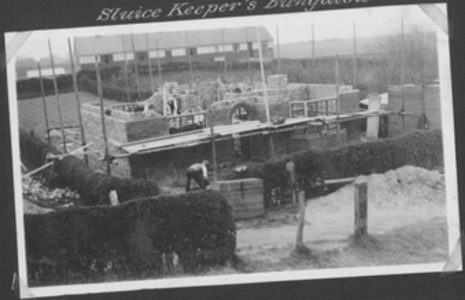
Building in Progress.
