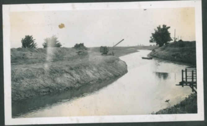
10 R.B. COMPLETING BED EXCAVATION.
