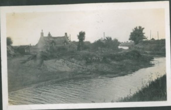
CORNER BEFORE WORK COMMENCED
