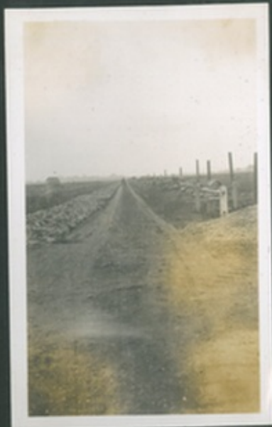
STONE PITCHING IN PROGRESS.
