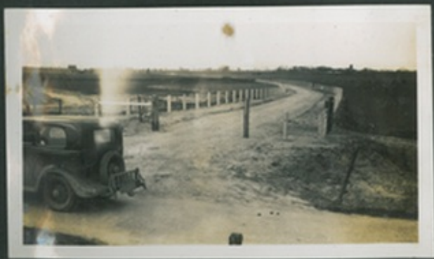
NEW ROAD COMPLETED.
