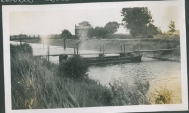
JOBSON'S BRIDGE RECONSTRUCTION. TEMPORARY BRIDGE AND WORK IN PROGRESS.
