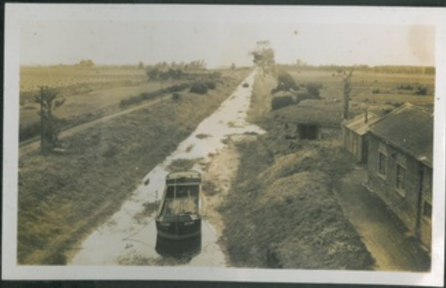
BEFORE FROM PODE HOLE ENGINE HOUSE.
