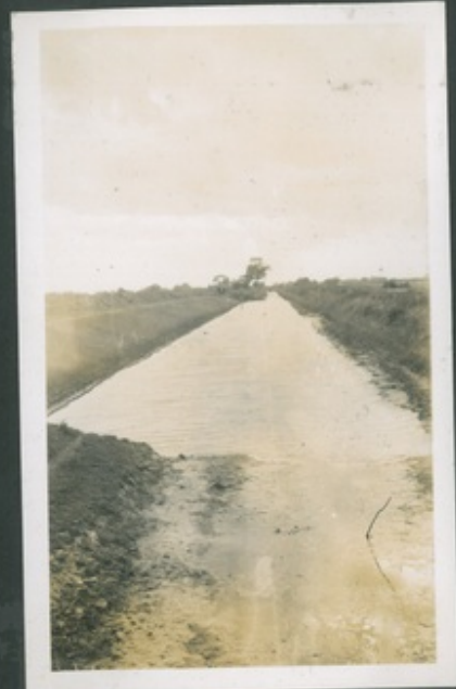
WORK IN PROGRESS LOOKING TOWARDS PODE HOLE FROM JOBSON'S BRIDGE.
