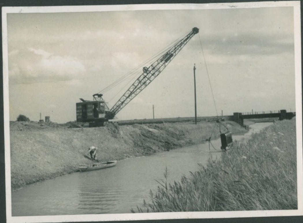
33 R.B. WORKING BETWEEN SHARP'S BR. AND RLY. BR. LEFT BANK.
