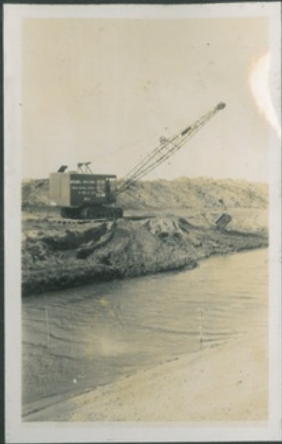
33 RB. IN HEAVY EXCAVATION
