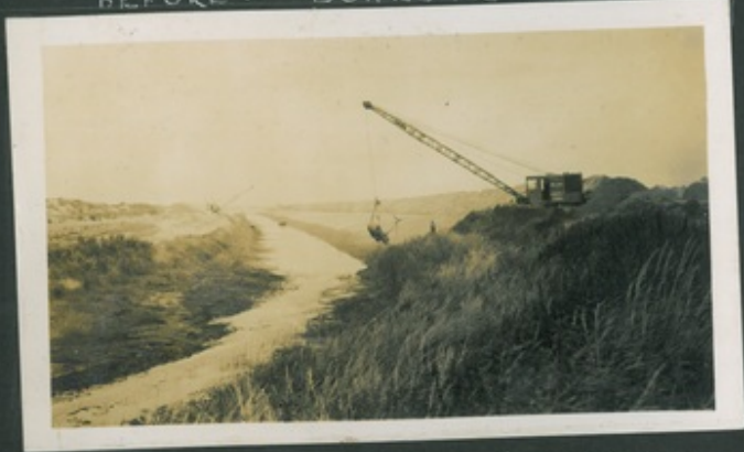
APPROACHING PLATT'S BRIDGE.
