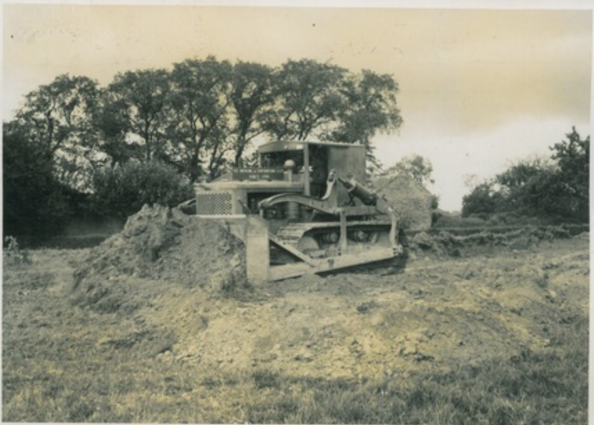
T. D. 18 HYDRAULIC BULLDOZER UPSTREAM SHARP'S BRIDGE RIGHT BANK.
