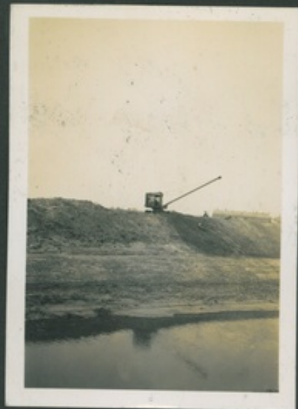
10 R. B. SHAPING SPOIL BANK.
