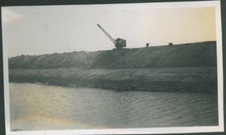
10 R.B. FINISHING SPOIL BANK.
