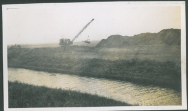
EXCAVATION FOR BERM.
