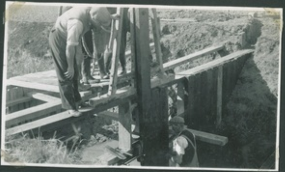
Pitching 9" x 5" Pile.
