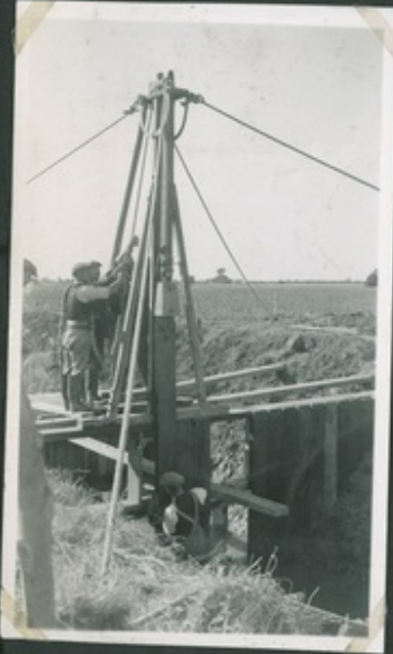
Pile Engine in action.
