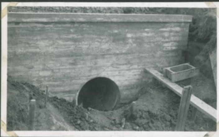
Shuttering removed. Wall drying-out.
