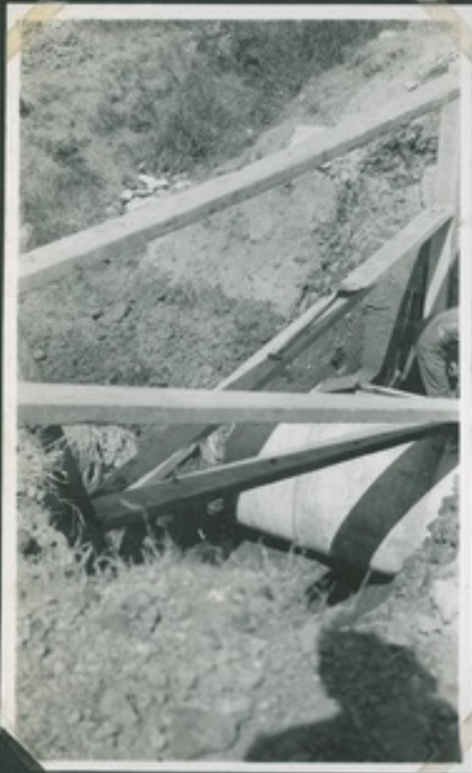
Preparing for Shuttering to Headwall.
