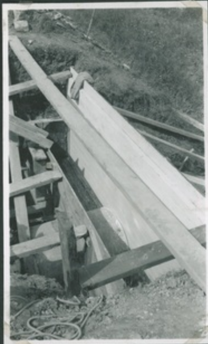
Shuttering in position for second step.
