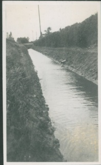
BOARD'S DRAIN 3 CHAINS FROM FLOODING NOTE - LAND PIPES.
