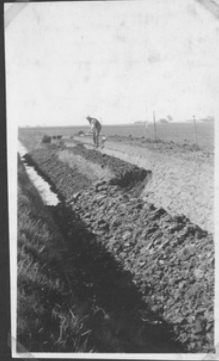
Colching opposite bank to Dragline.
