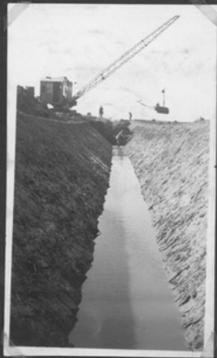
Work in Progress.
