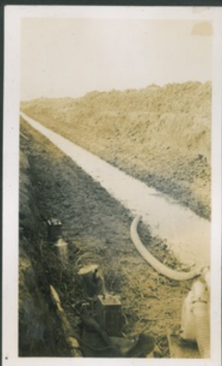
TOE PILING COMPLETED - FAGGOTTING IN PROGRESS.
