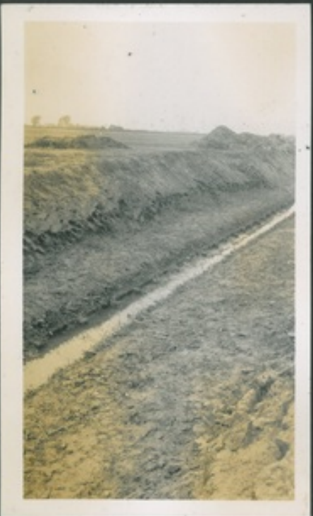
TOE PILING COMPLETED - FAGGOTTING IN PROGRESS.
