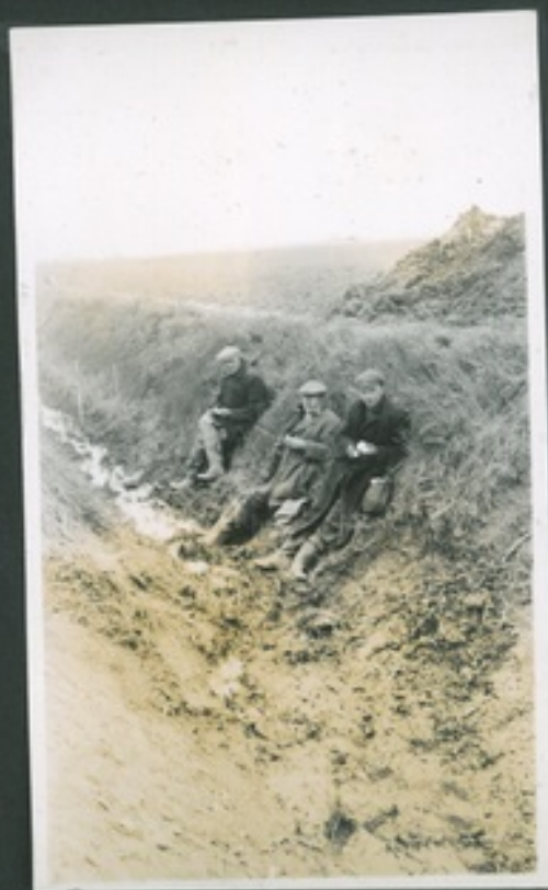
Existing Drain & Gang.
