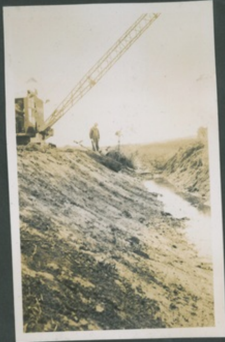
WORK IN PROGRESS NOTE - FALL FROM OLD FANTAIL INTO NEW DIVERSION.
