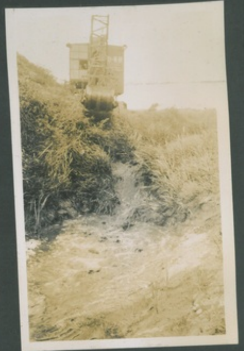
WORK IN PROGRESS NOTE - FALL FROM OLD FANTAIL INTO NEW DIVERSION.
