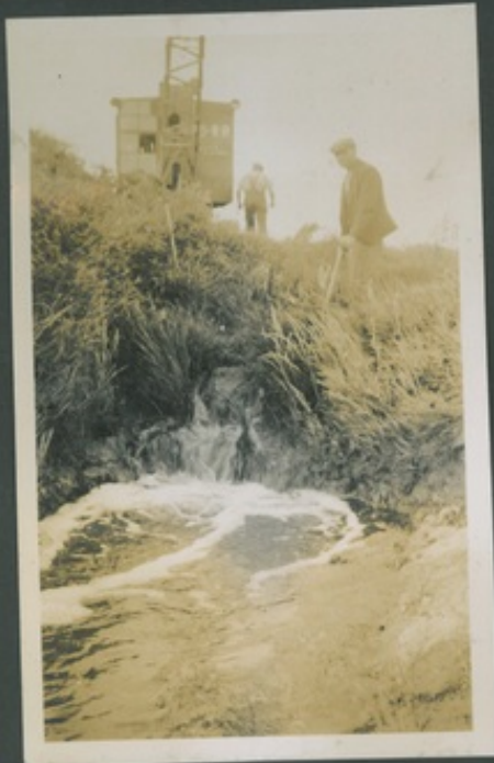
WORK IN PROGRESS NOTE - FALL FROM OLD FANTAIL INTO NEW DIVERSION.
