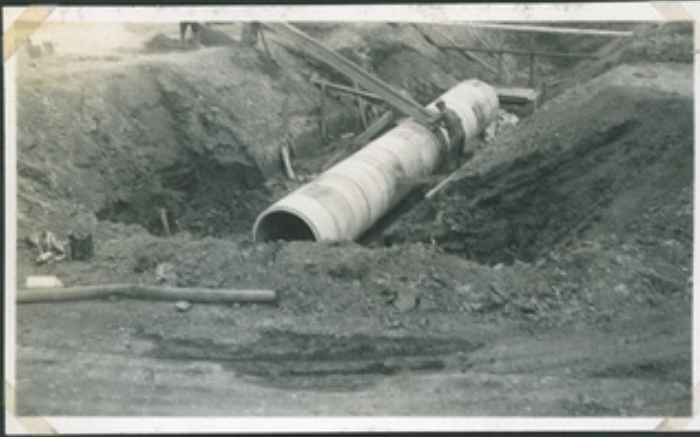
CONCRETE PIPES LAYED HAUNCHING IN PROGRESS.
