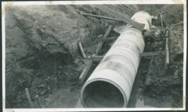
CONCRETE PIPES LAYED HAUNCHING IN PROGRESS.
