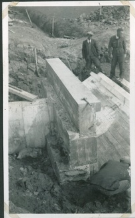
REMOVAL OF SHUTTERING FROM HEAD WALL.
