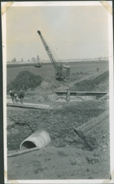
TEMPORARY ROAD OVER.
