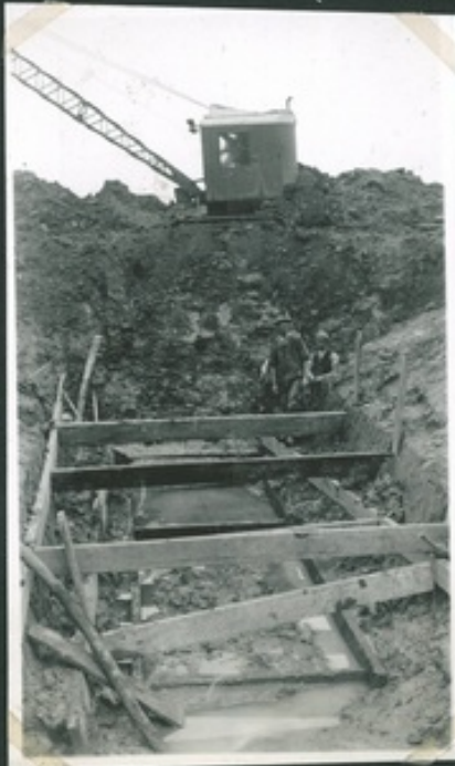
LAYING CONCRETE FOUNDATION AFTER PILING.
