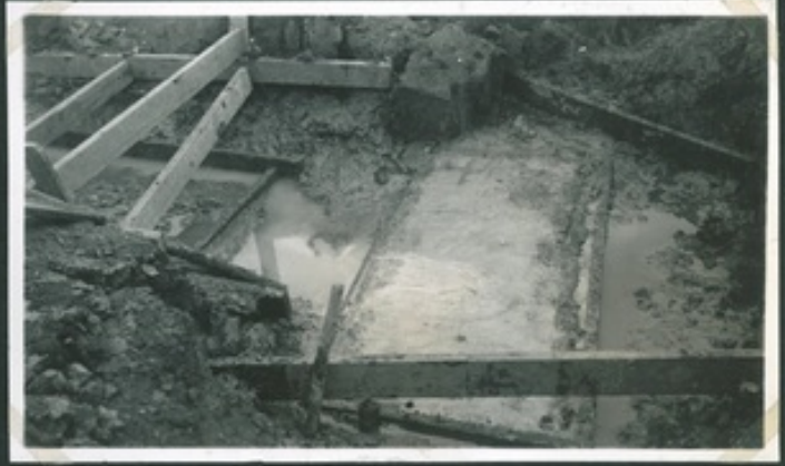
CONCRETE FOUNDATION FOR HEADING WALL
