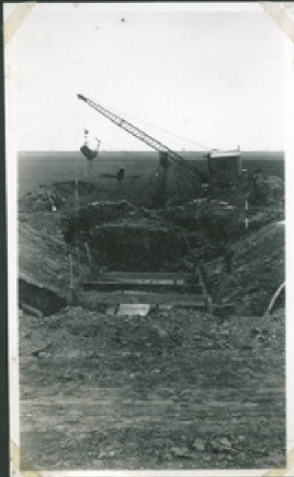
LAYING CONCRETE FOUNDATION AFTER PILING.
