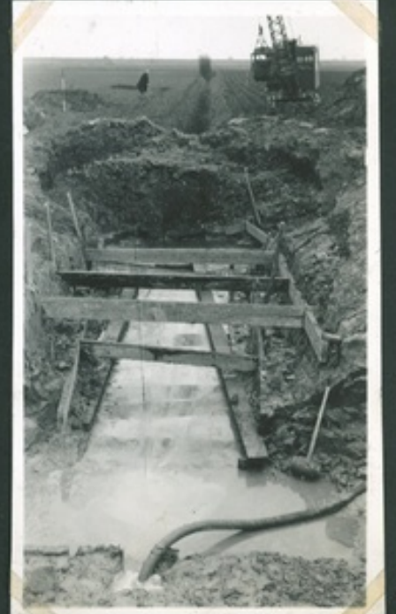
LAYING CONCRETE FOUNDATION AFTER PILING.
