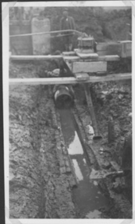
LAYING NEW CONCRETE PIPES.
