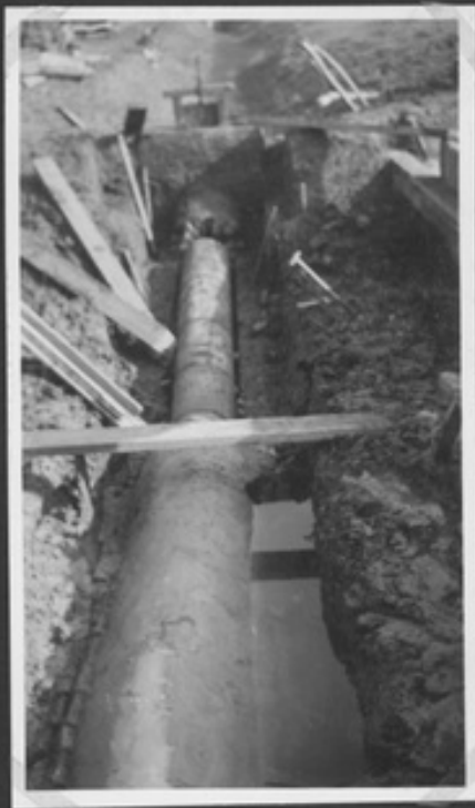
CONCRETE HAUNCHING IN PROGRESS.
