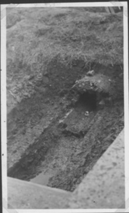
DEMOLITION OF OLD TUNNEL.
