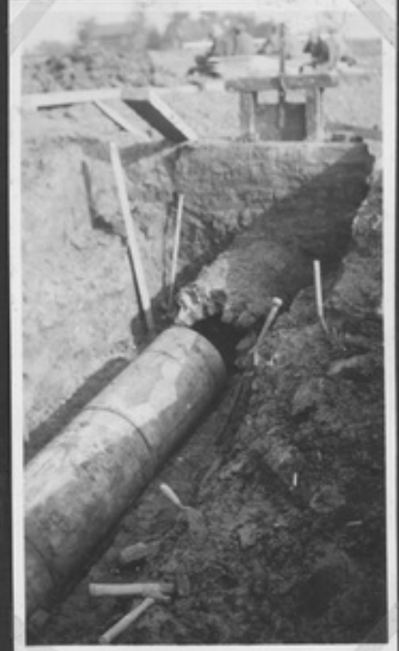
LAYING NEW CONCRETE PIPES.
