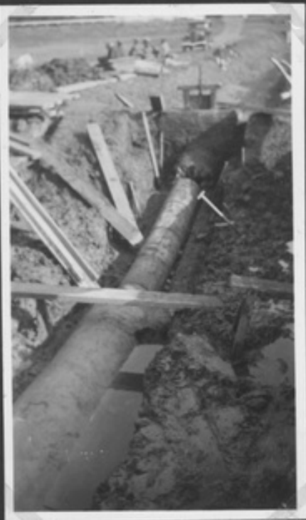
CONCRETE HAUNCHING IN PROGRESS.
