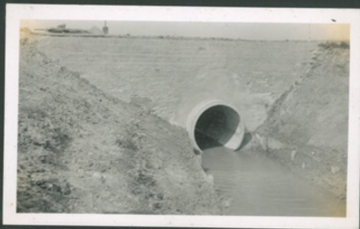
Repair of Culvert.
