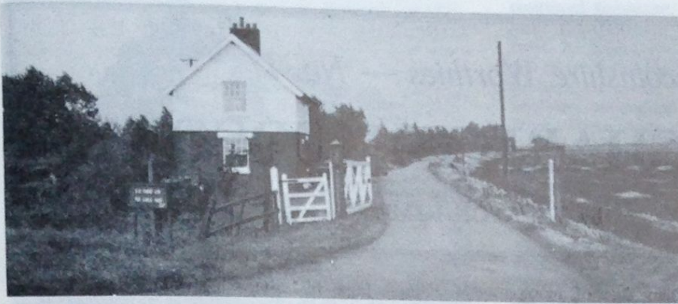
Left: Once Counter Drain railway station, now The Earl's Farm.
