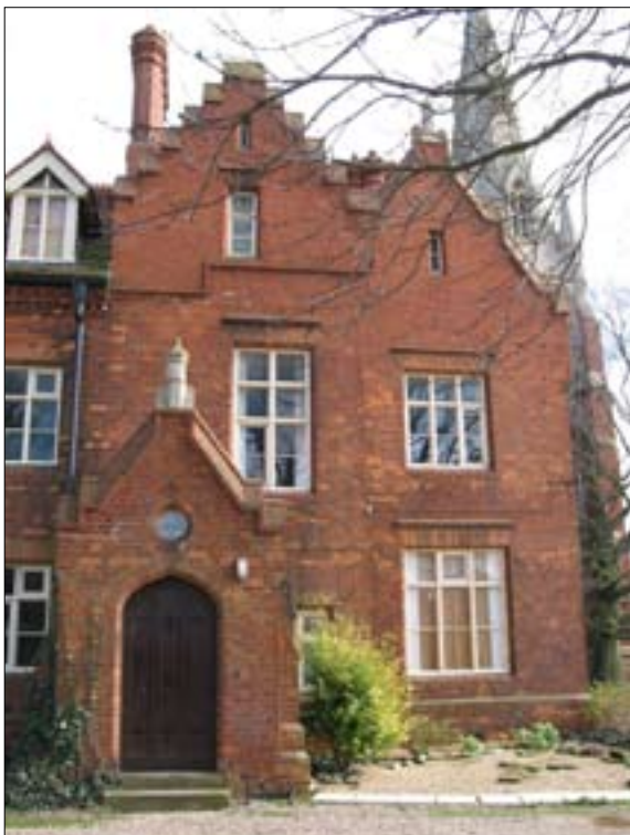
Fig. 12. The vicarage, west elevation. © John Minnis 2007
