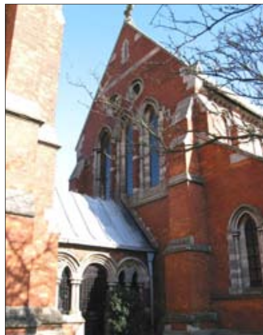
Fig. 3. Passage between the tower and the nave. © John Minnis 2007
