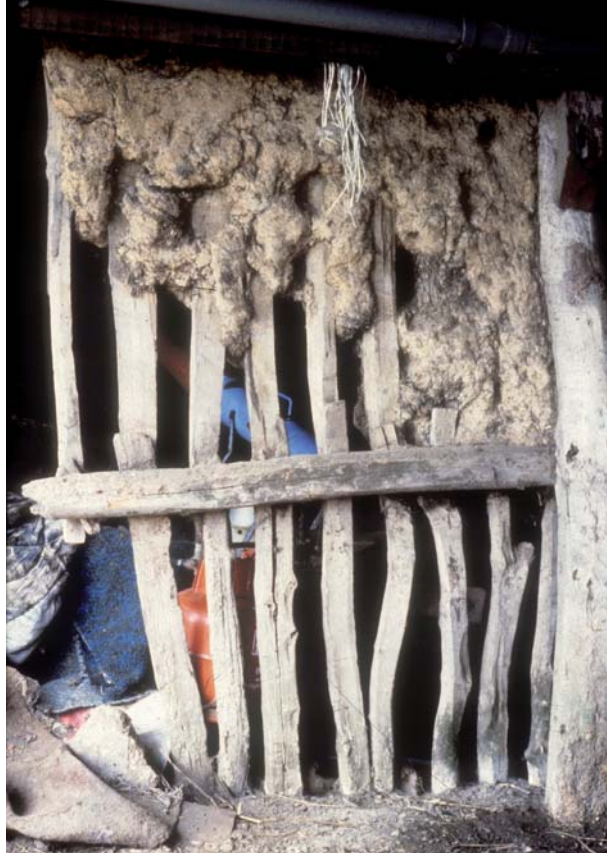
Decayed mud and stud wall in a barn in Gosberton (1983)
